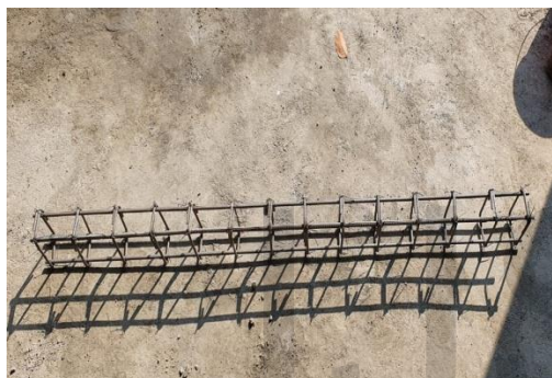
Figure 5 : Reinforcement bars tied with stirrups
